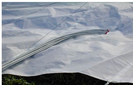
Working from the centre outwards, insert the upper surface battens.
